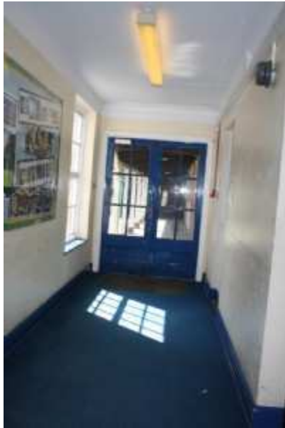
Inner Main Entrance Lobby with Staff Room on the Right
