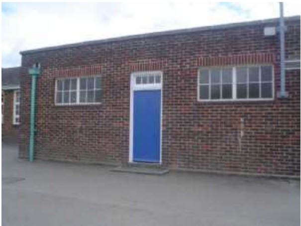
The Sports Changing Room and Shower Block.
